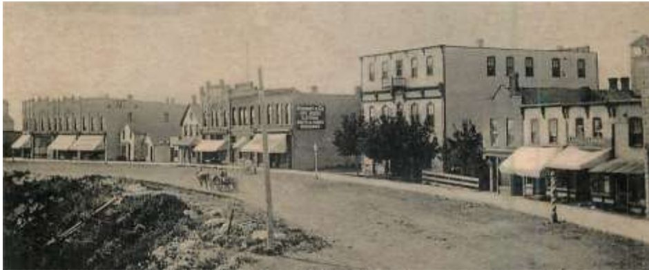
Crescent Avenue in the early 1900's
